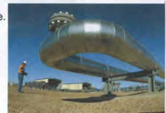
Fracking requires industrial drilling infrastructure
